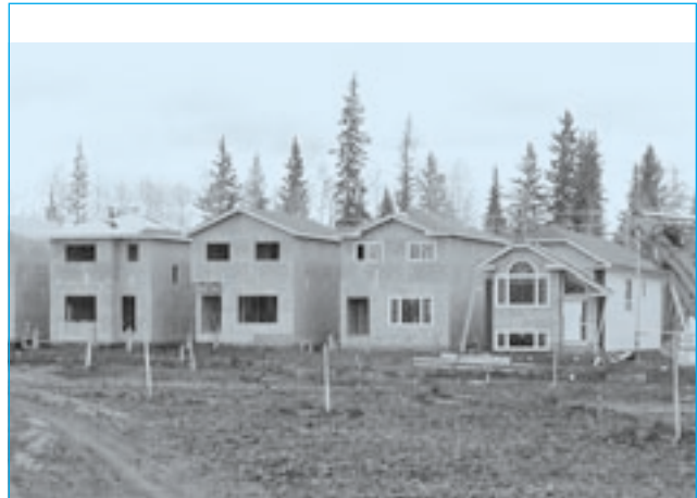
NewNorth construction, Fort McMurray, AB
