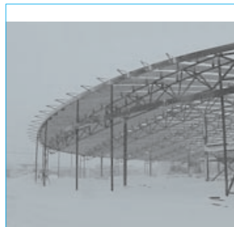
Cambridge Bay School structural steel, NWT
